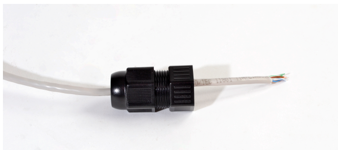
Figure 19 – Fastening the plastic counterpart to the cable
